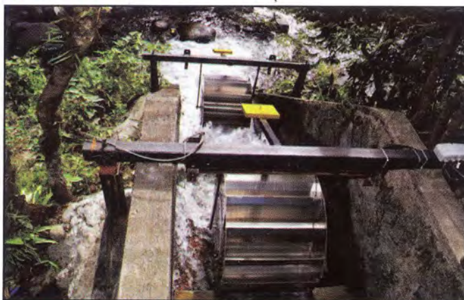
The first picohydro system in the country built and installed in Southern Leyte is expected to generate power up to 600 W.
